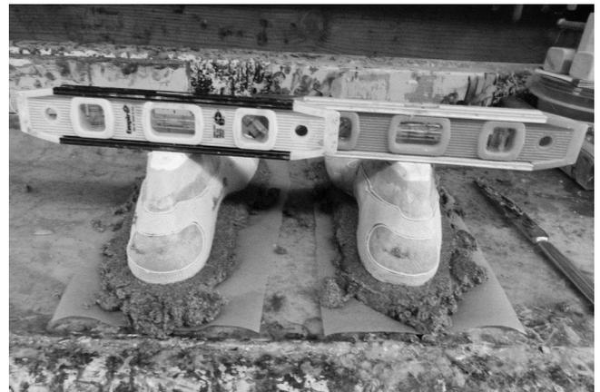
54 Both levels were checked as the "mud" was pressed down to the design cords.
